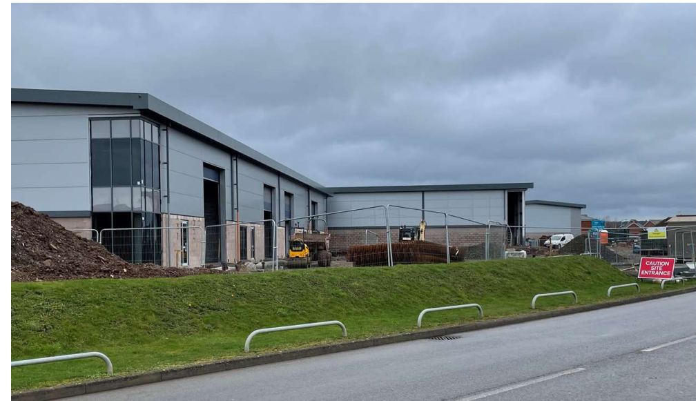
Construction opposite site
